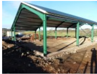
Roof panels on Jan 2017
