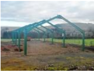
Steel frame erected Nov 2016
