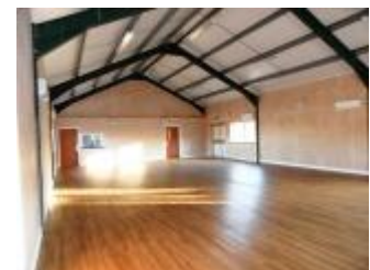
Hall floor laid Feb 2018
