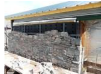
Stonework for entry porch built April 2017
