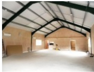
Concrete floor laid and interior wall constructed June 2017
