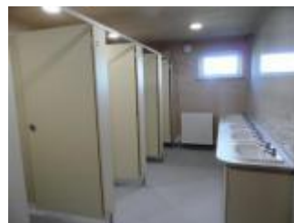
Ladies toilets June 2017
