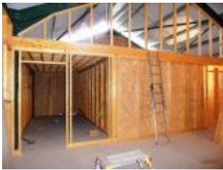
Partition walls for kitchen and Toilets built Feb 2017
