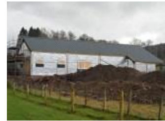
Infill panels with insulation Feb 2107
